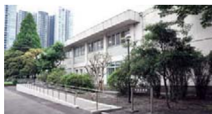
附属図書館 (本館) University Library (Main Library)
