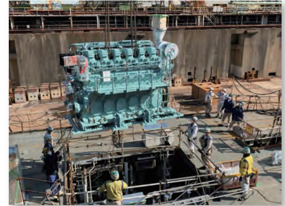
主機搭載 Installation of main engine
